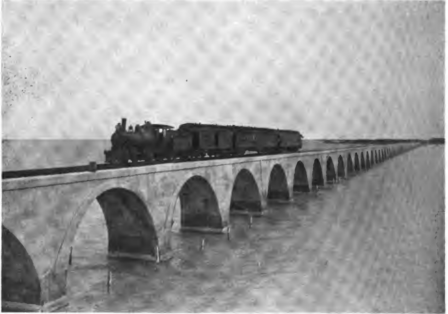
Long Key Viaduct. —Total distance between abutments at the springing line, 10,444.65 feet; 181 piers; 180 arches; additional water opening Long Key to Grassy Key (embankment) 19,100 feet; total opening Long Key to Grassy Key, 29,544.65 or 5.6 miles.
